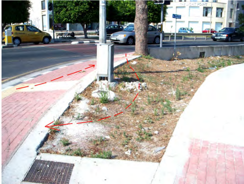
Figure 2.8: Existing footway at Nea Engomi Street junction
