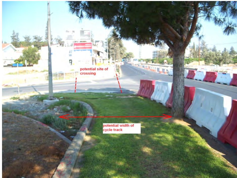
Figure 2: Junction at Grigori Afxentiou (looking east)
