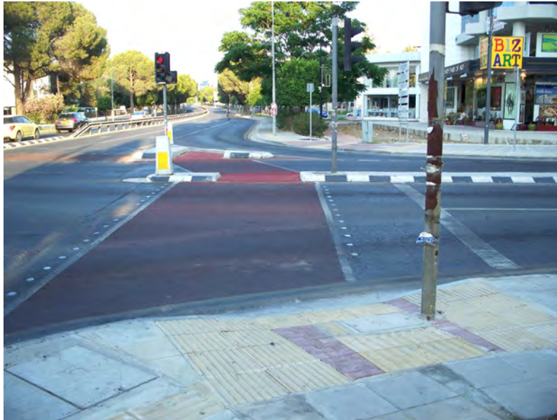
Figure 2.6: October 28th Street junction with Grivas Digenis Avenue
