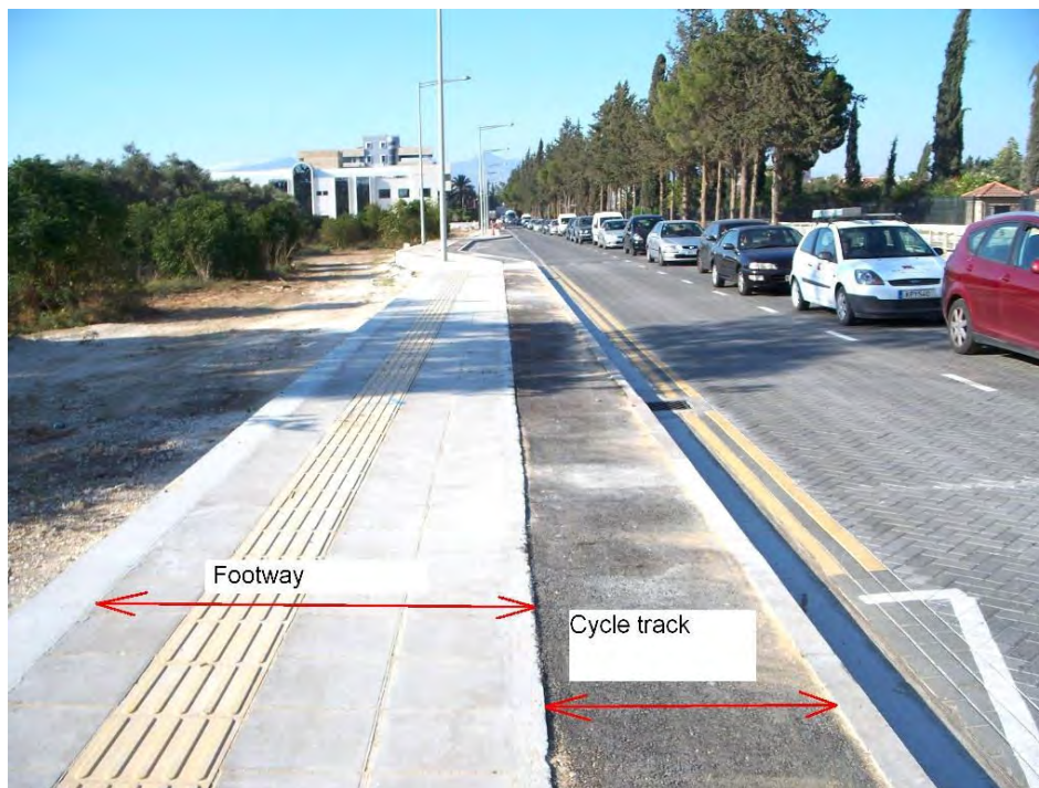
Figure 1: New pavement laid as part of Archangelou works incorporating cycle track (Agios Prokopiou looking north)
